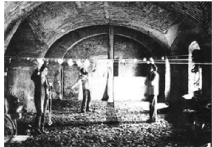
SHEAR ROOM BEFORE ITS RESTAURATION
